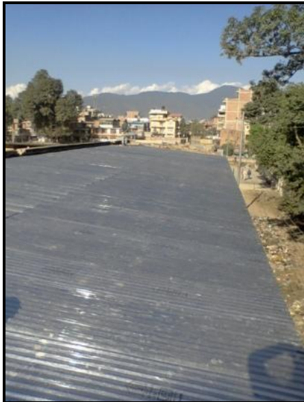
New roofing iron
